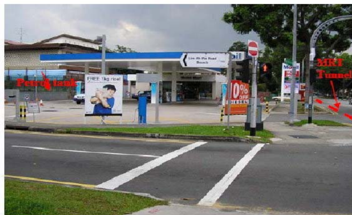
Underground fuel storage tanks outside 1 st reserve. Tanks and associated piping equipped with automatic leak detection and monitoring system
